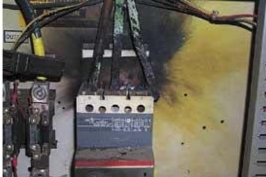
*Fig. 4: Loose input power connections*
