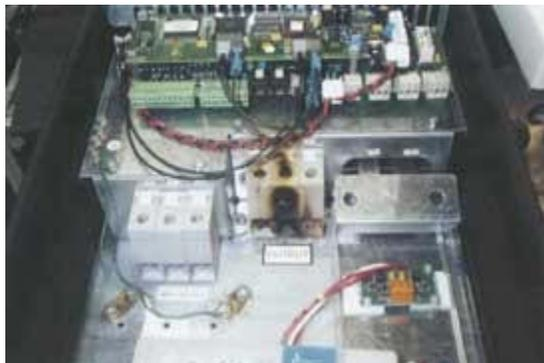
*Fig. 5: Loose output power connections*
