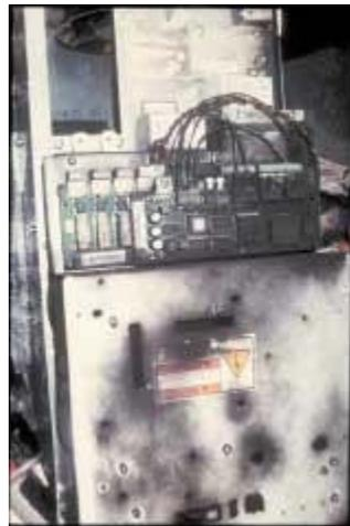
*Fig. 2: Fan injecting dust particles into VFD.*
